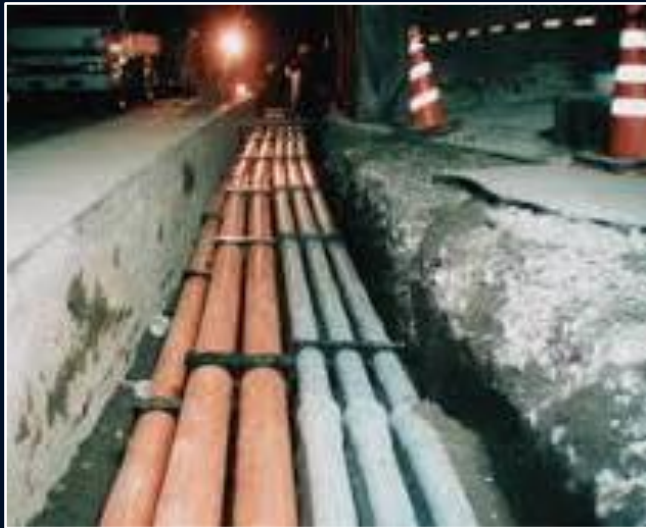
"Promote boosts to the disappearance of utility poles" Object: CCVP pipe (Power cable protection tube) (Orange) Object: ECVP pipe (General PVC pipe) (grey)
