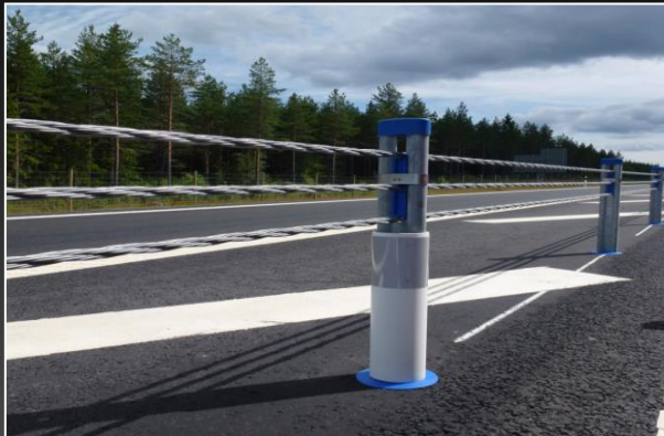
Wire rope type protective fence for overseas expressway road shoulders ・ As visual guidance of road, 2,500 km provisional two-lane guard fences nationwide, Guide path guidance at earthquake disaster, Overseas highway guard fences, Road shoulder blocks in developing countries
