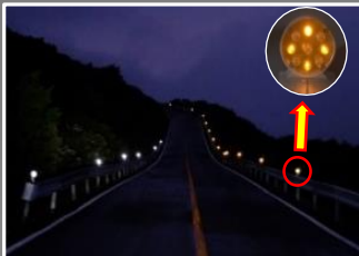
Recognition of "points" by existing type delineator 3 . Even when a car collides, it will not scatter to the opposite lane and prevent secondary accident
