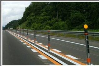
A wire rope type protection fence that can prevent the vehicle from jumping out but it has poor visibility
