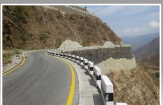
As a safety measure for the Road Shoulder Block of Developing Countries
